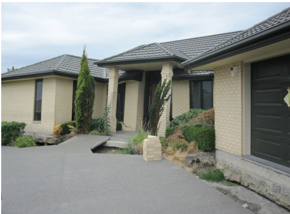
Figure 5. Typical liquefaction damage to modern single-family home in Christchurch, New Zealand. Note that this home will likely need to be completely rebuilt due to extensive foundation damage.
